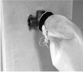
13. Next, cover the faucet with the bag provided in order to protect the faucet while the wall is finished off. Make sure that no dust can reach the faucet.
